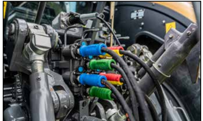
Fig. 25 Hydraulic Circuits Installed
