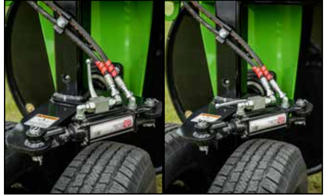
Fig. 47 Steering Circuit Hydraulic Ball Valves: Closed/Open
