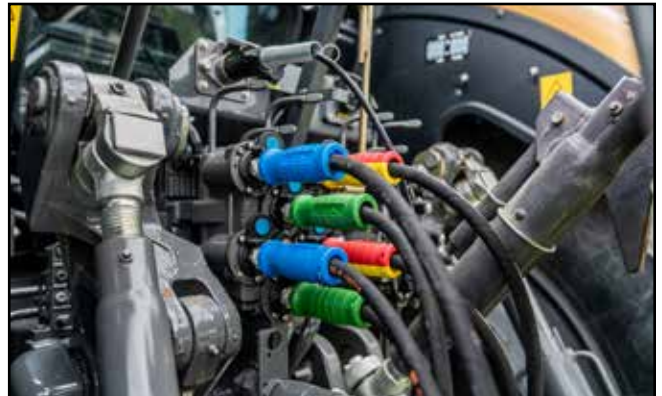
Fig. 25 Hydraulic Circuits Installed
